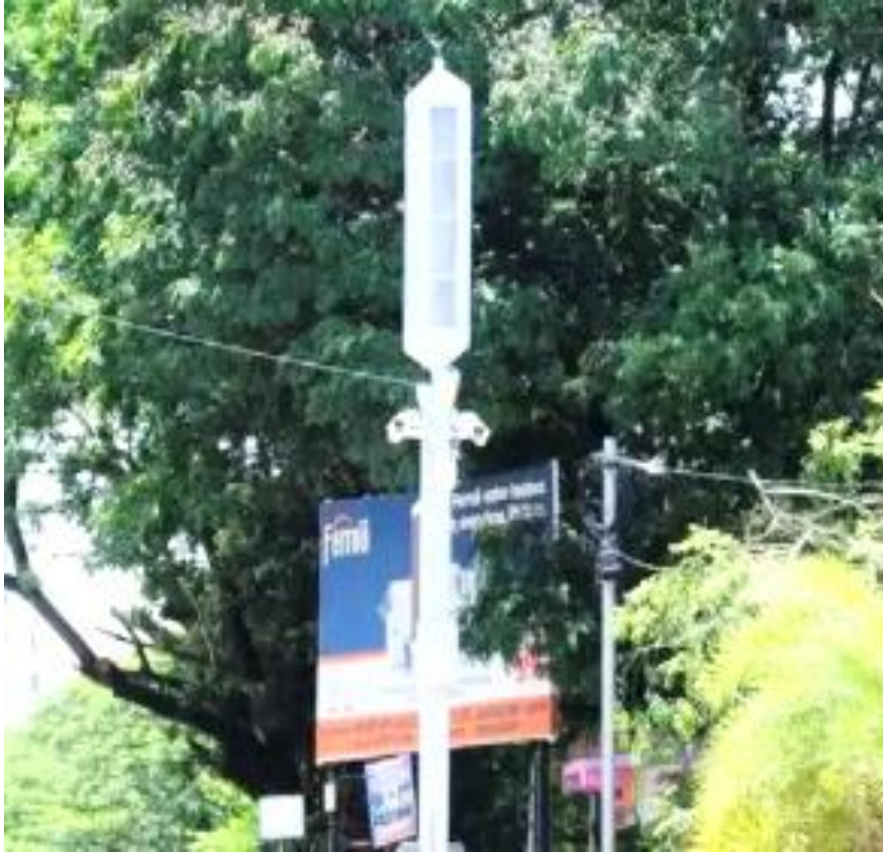
Smart Poles, Mangaluru
