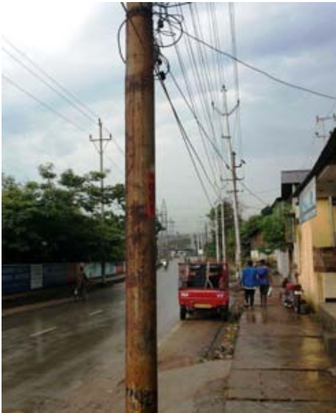
33 kV line inside city area of Assam
